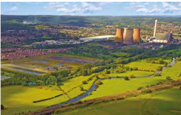
Rugeley Power Station, which has been decommissioned, provides significant potential for regeneration
